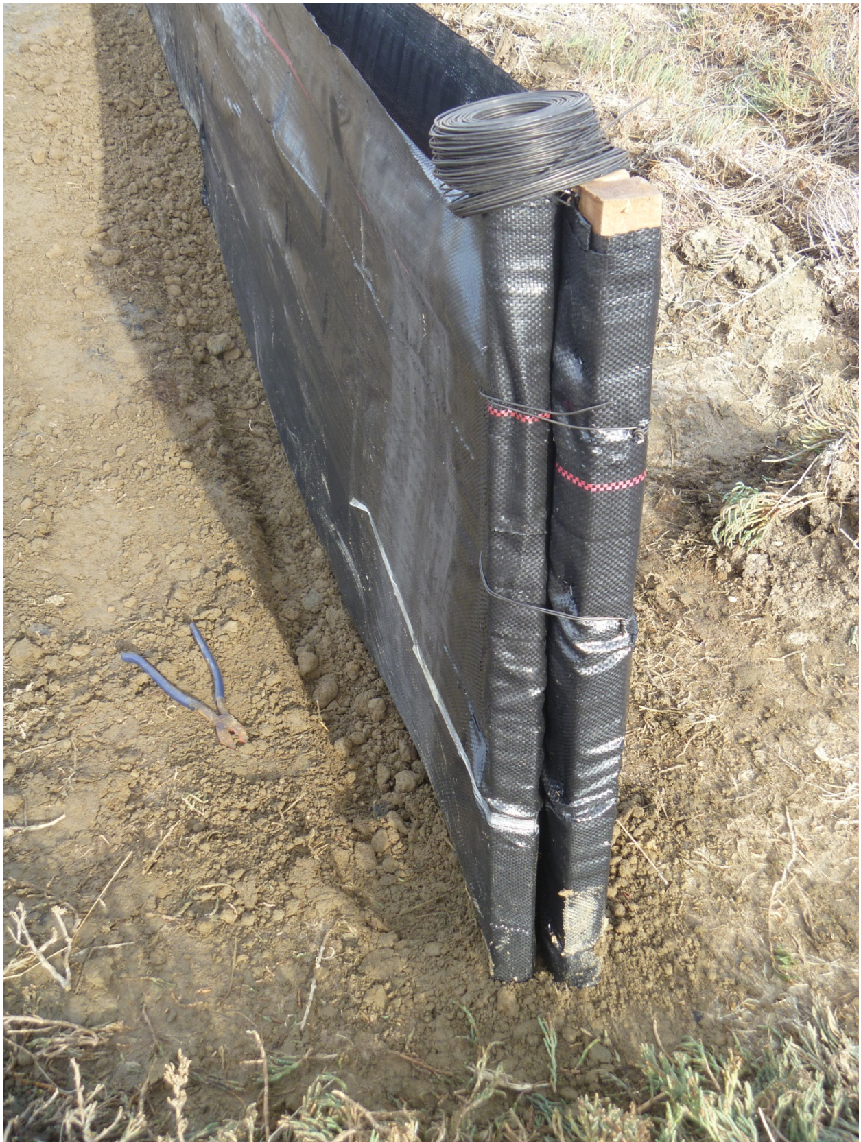
South end double wall silt fence. West side 8-acre FSFA.
