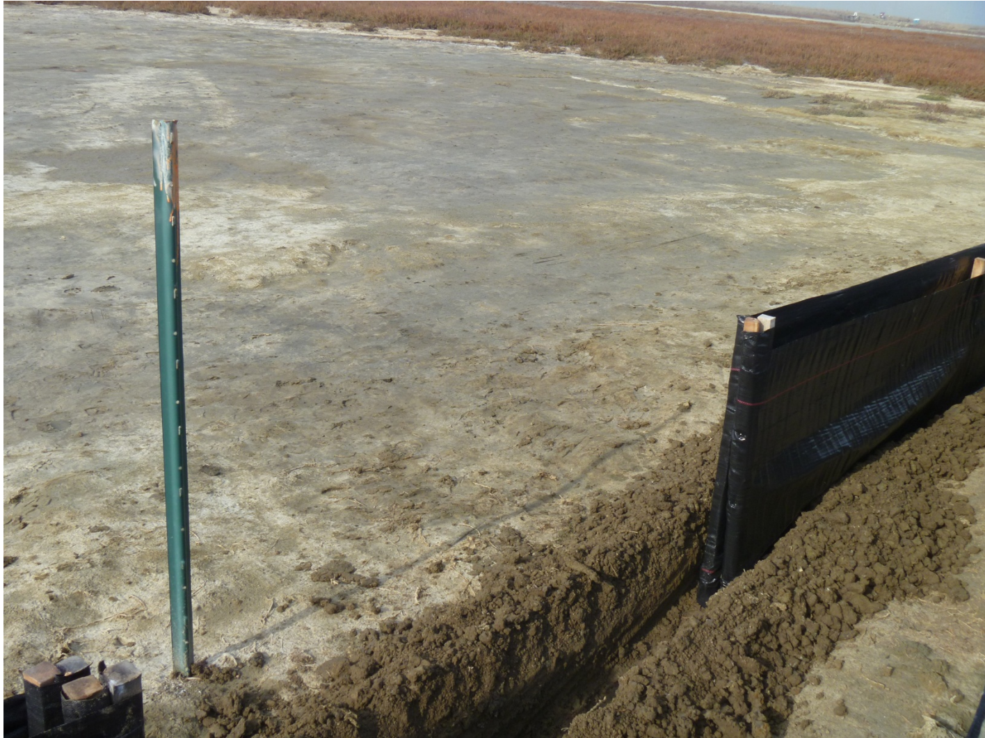
ICAM sample location SDS03. Silt fence and trench.
