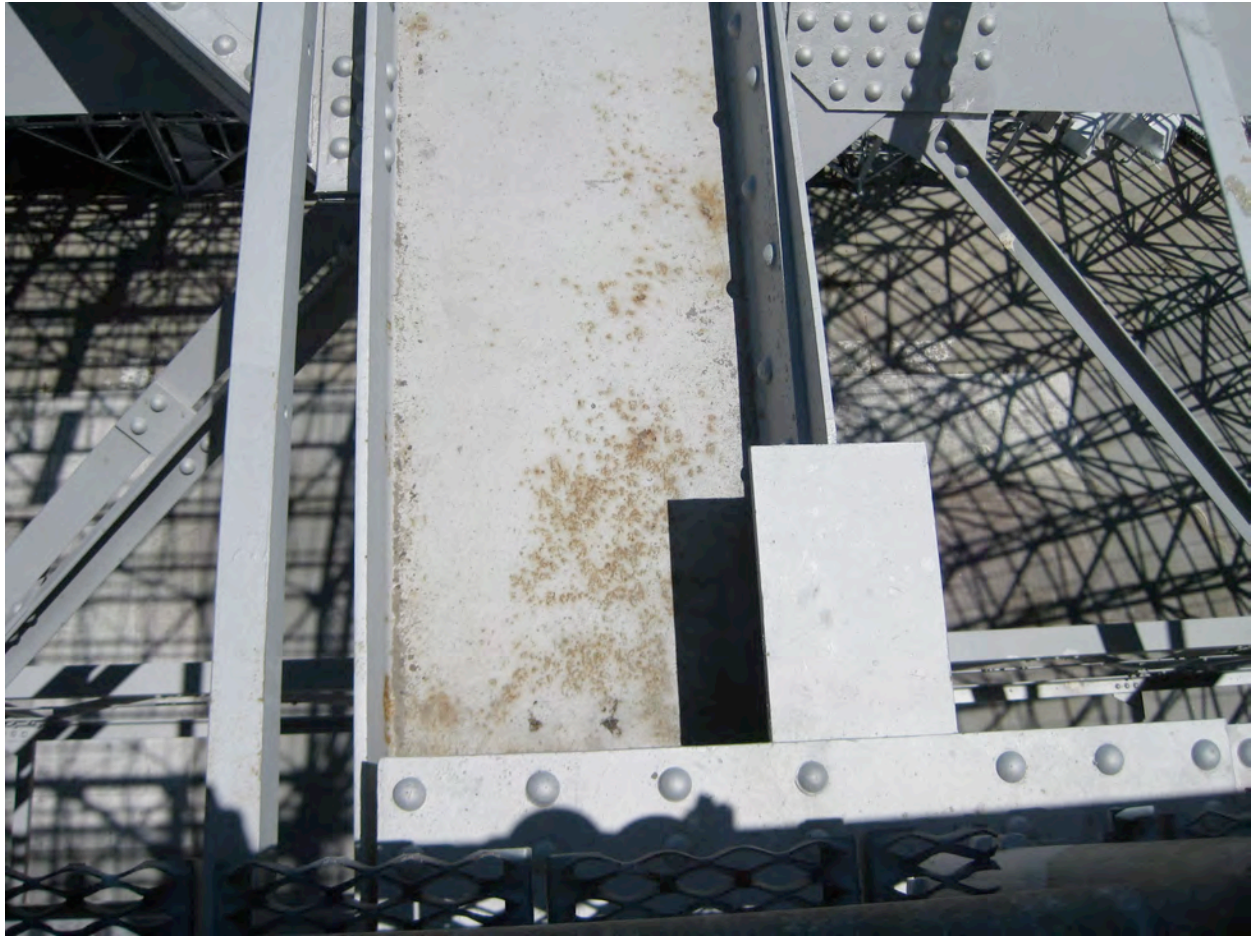
Roof-top rusting of NTCRA Coating
