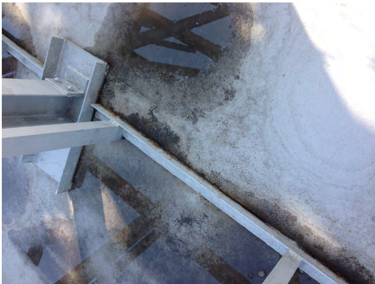
Mezzanine Pooling Water & Sediment
