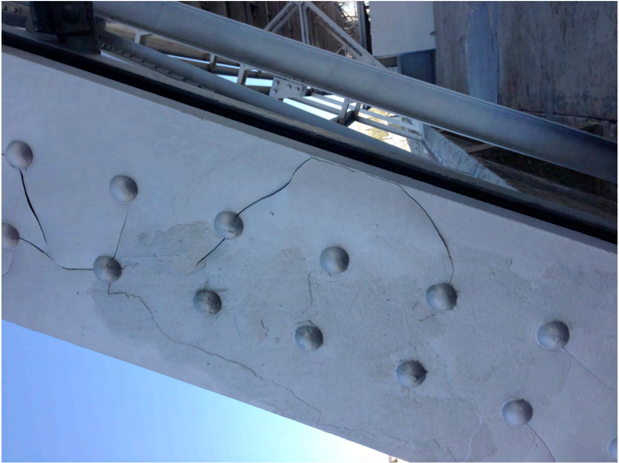
Delaminating encapsulant and original paint, vertical steel
