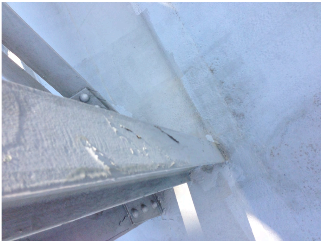
Peeling Edges of Original Coating, vertical steel
