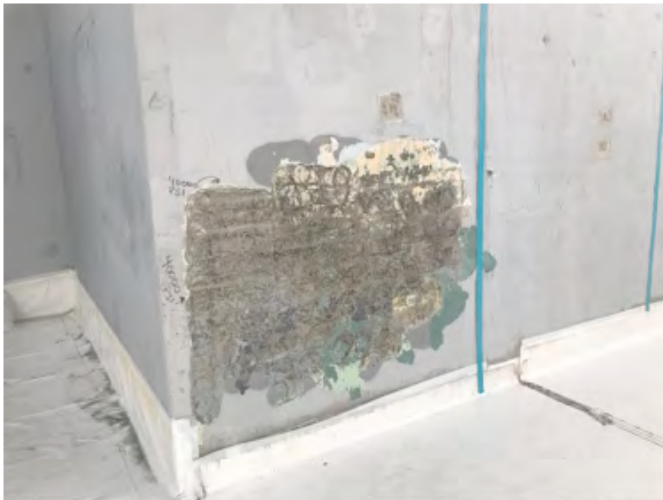
Photograph 6 – CMU wall after removal of paint/coatings with UHPW system.
