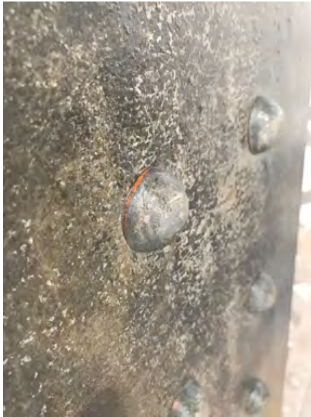
Photograph 3 – Primer evident around rivet head after UHPW removal.
