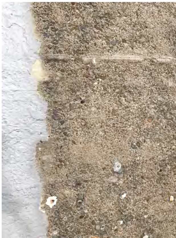
Photograph 18 – CMU wall after removal of paint/coatings with vapor media system.
