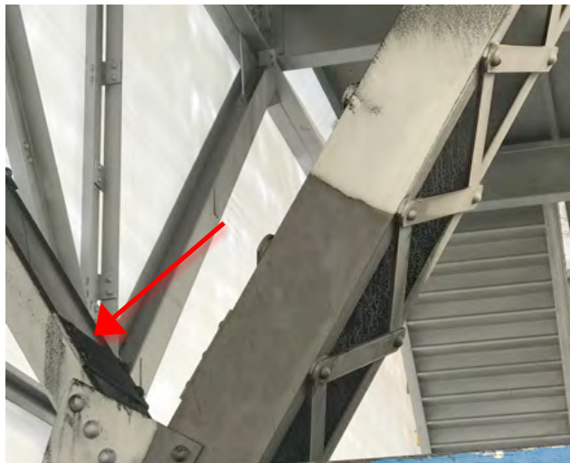
Photograph 14 – Structural steel after removal of paint/coatings by vapor media system. This photo was taken before cleaning the Pilot Study enclosure and black areas (see the red arrow) are areas where spent abrasive media has accumulated.
