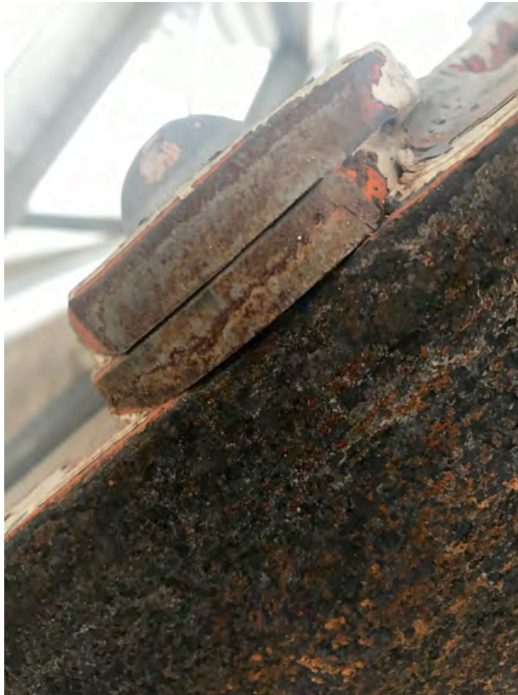
Photograph 1 – Structural Steel after abatement with UHPW. Note the presence of black mill scale, paint/coatings in tight-tolerance mated surfaces and rough surfaces.
