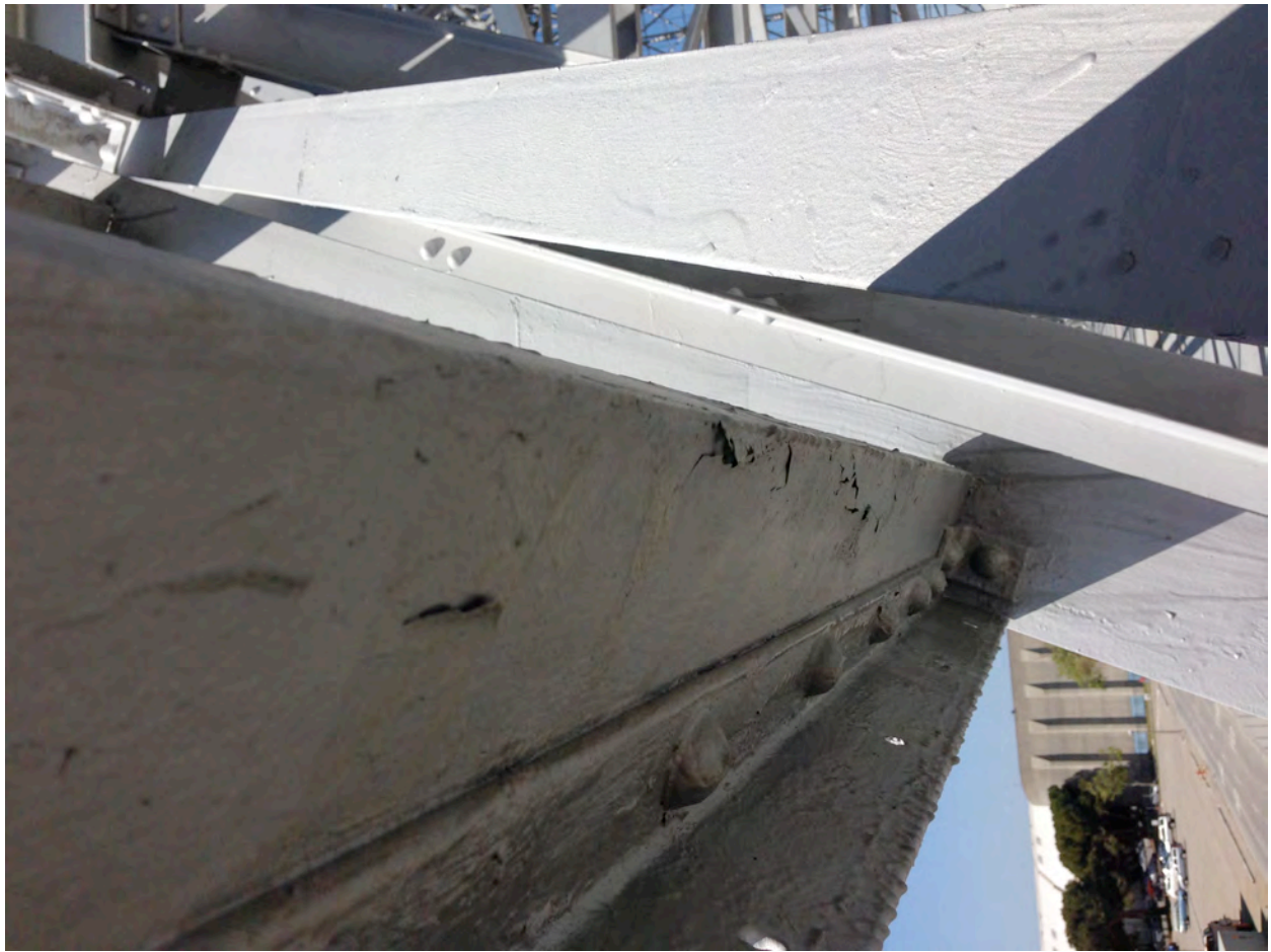
Loose & peeling original coatings, horizontal steel
