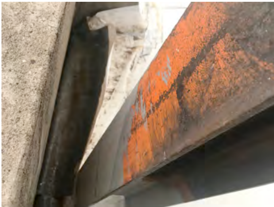
Photograph 4 – Poor removal of paint/coatings where UHPW nozzle was difficult to aim in tight access areas.
