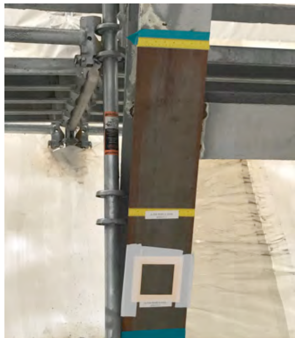
Photograph 16 – Structural steel after removal of paint/coatings with vapor media system at time of verification sampling. Note the formation of surface rust.
