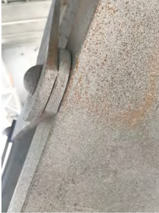
Photograph 10 – Structural steel with tight-tolerance mated brace and rivet head after removal of paint/coatings with media blasting. (Note: the brown areas in the photo correspond to areas of rust formation due to the wet decontamination of the abated steel)
