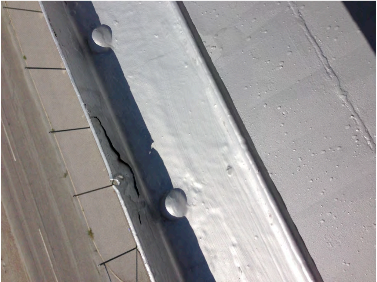
Delaminating encapsulant, horizontal steel
