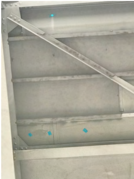
Photograph 11 – Under side of mezzanine after removal of paint/coatings with media blasting.
