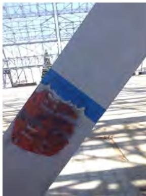
After Recoating/Repairs by DPR
