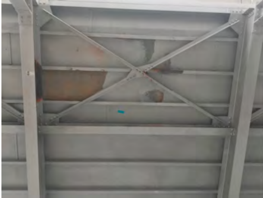
Photograph 5 – Underside of mezzanine after UHPW method was utilized.
