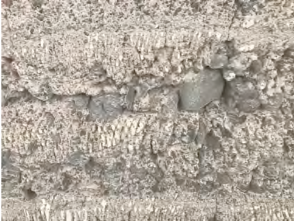
Photograph 7 – Damage to concrete and paint/coatings remaining on surface of CMU wall.
