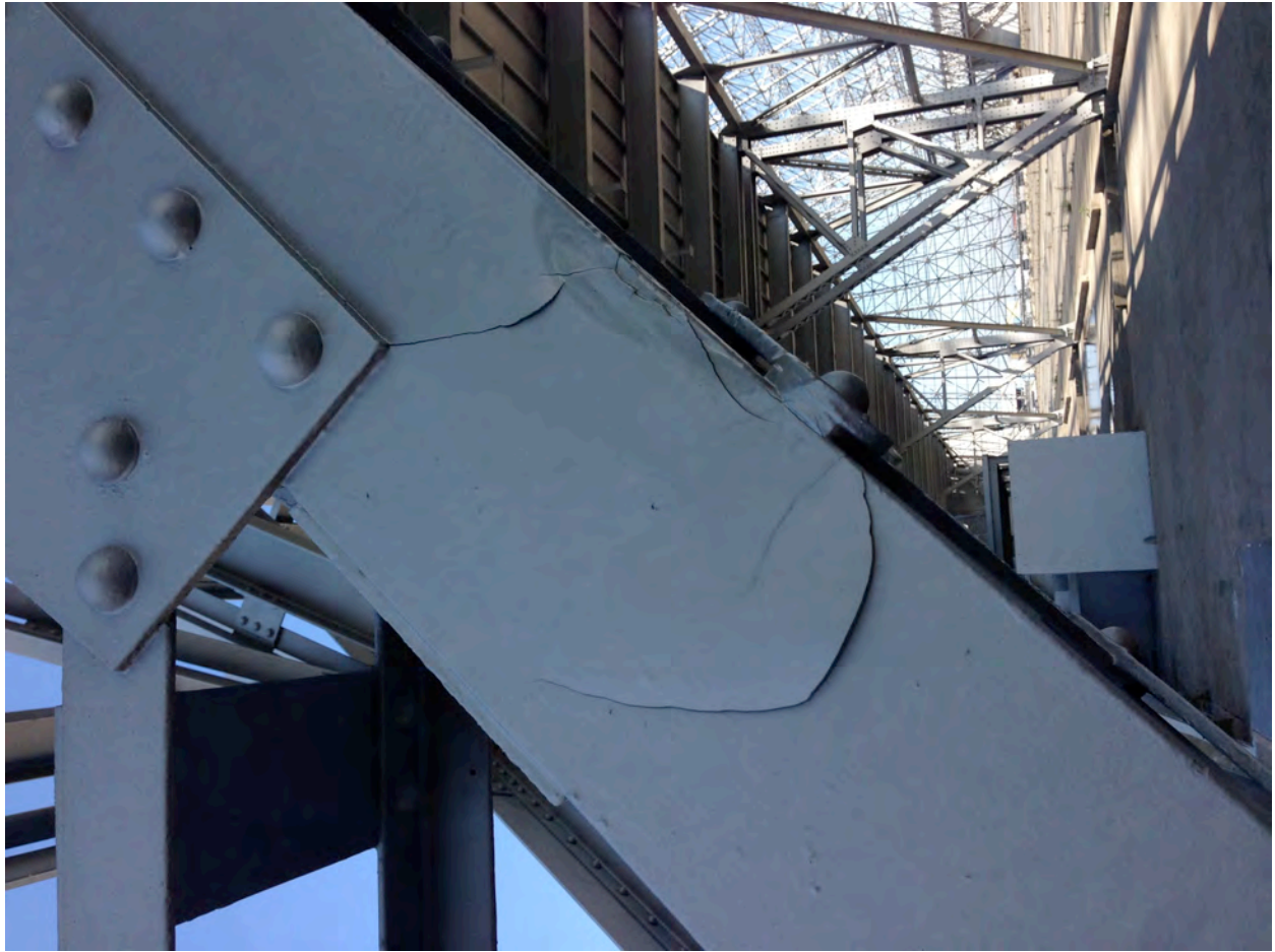
Delaminating encapsulant and original paint, vertical steel
