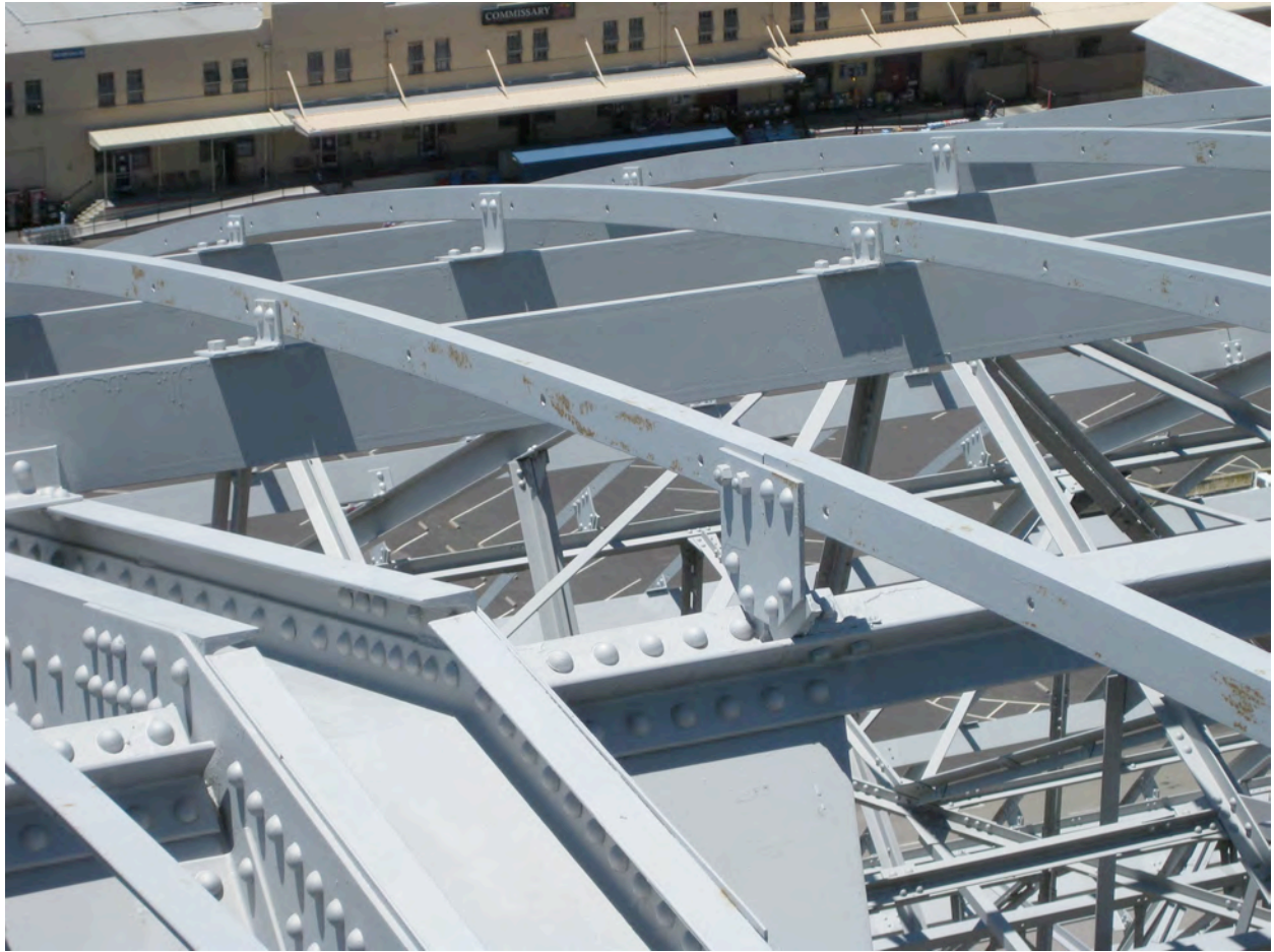
Roof-top rusting of NTCRA Coating
