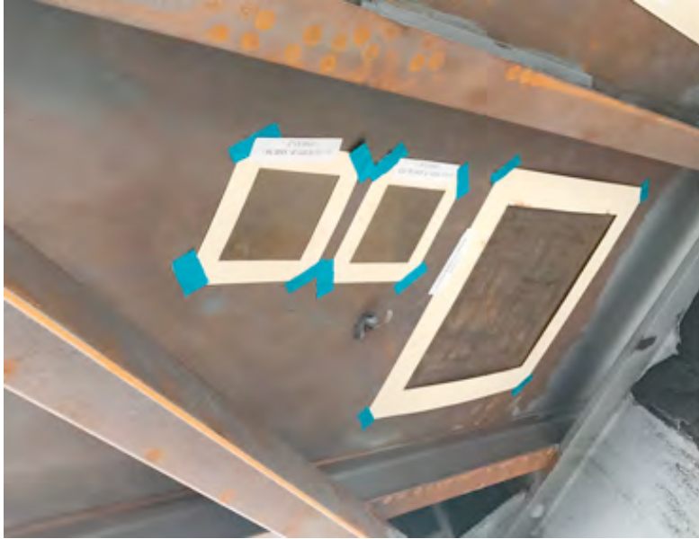
Photograph 17 – Under side of mezzanine after removal of paint/coatings at time of verification sampling. Note the formation of surface rust.
