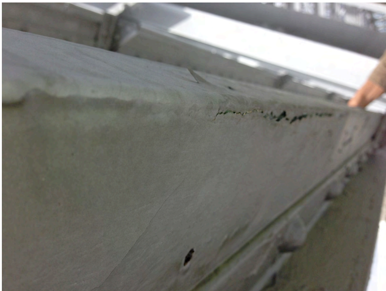
Deteriorated paint, underside of horizontal steel
