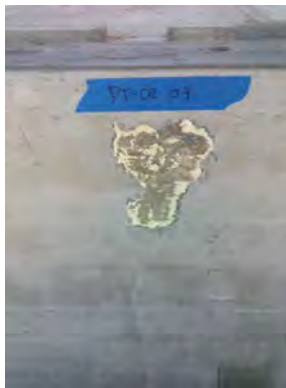
After Recoating/Repairs by DPR
