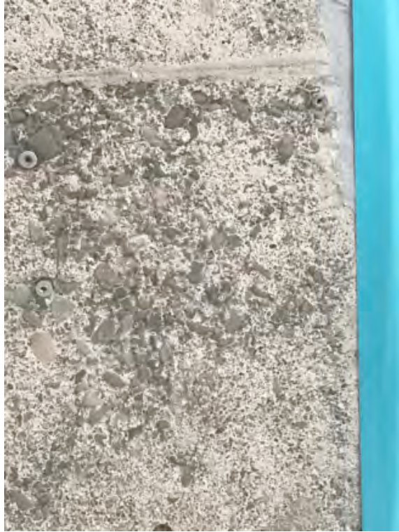
Photograph 13 – CMU wall after removal of paint/coatings by plastic bead media blasting. Removal method exposes aggregate and caused minor damage to “board form” markings on the CMU wall.
