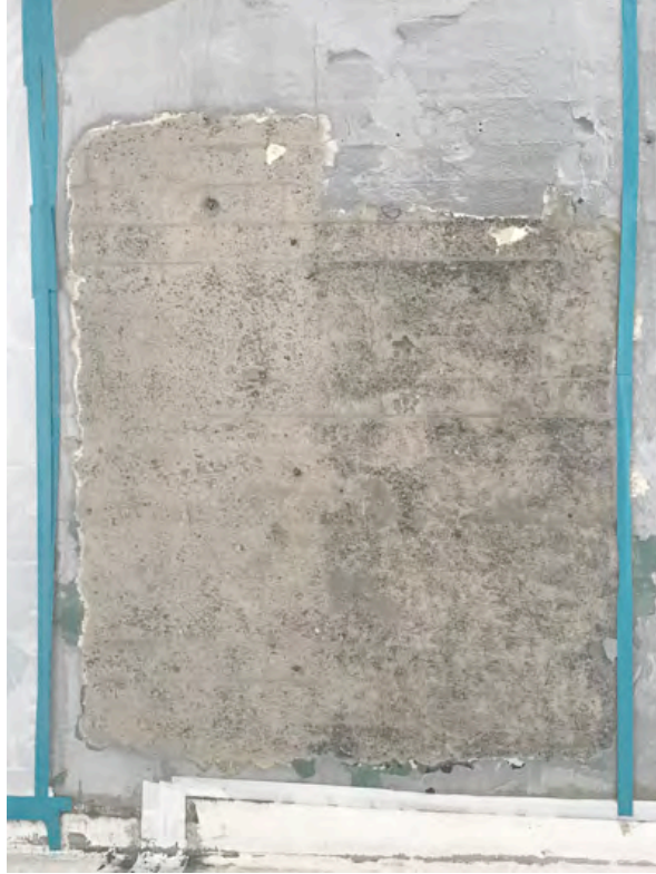
Photograph 12 – CMU wall after removal of paint/coatings with media blasting. Left side (lighter color) was removed with Kleen blast media. Right side (darker color) was removed using plastic media.
