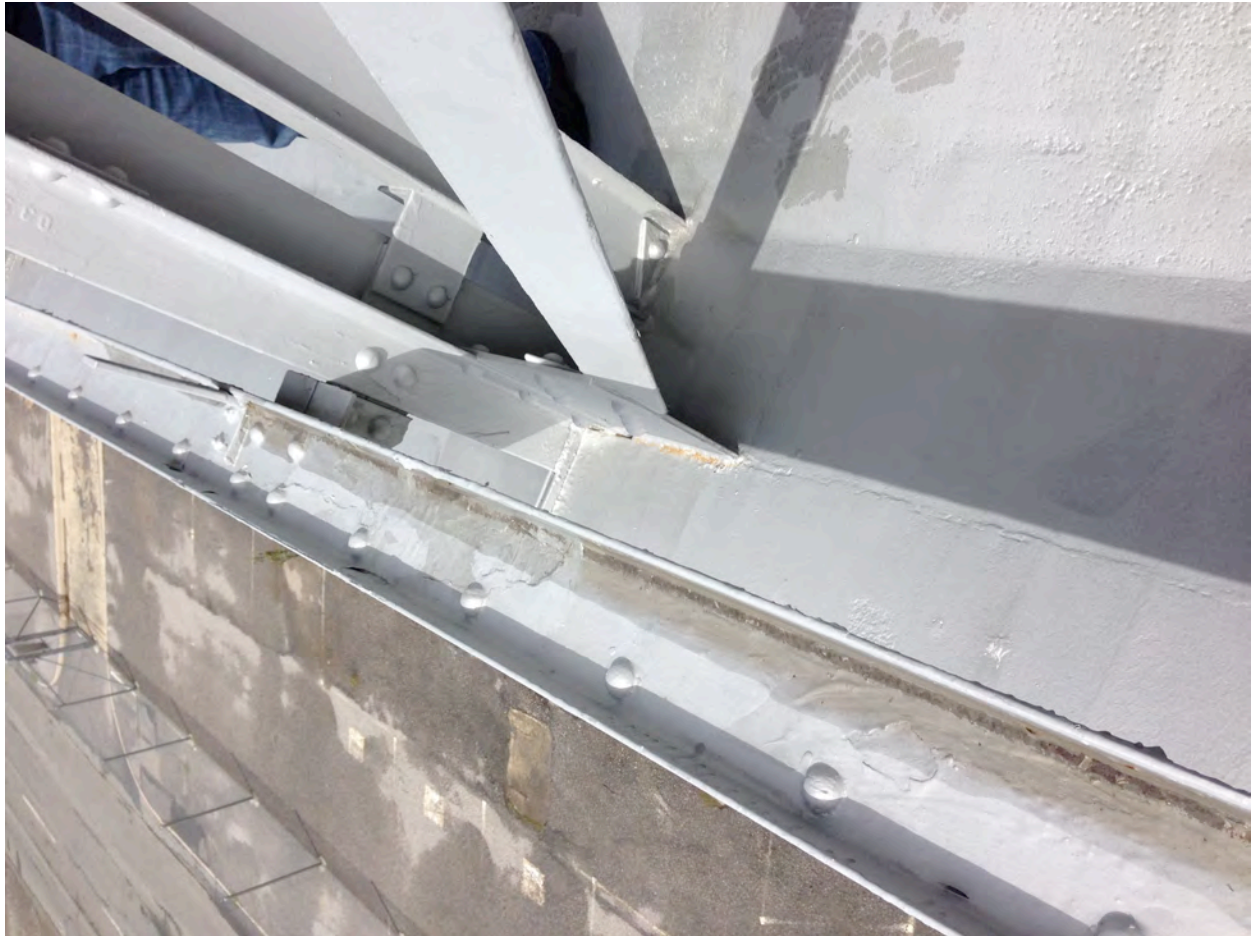
Pooled Water & Deteriorating Paint Edges (Horizontal Steel Framing)
