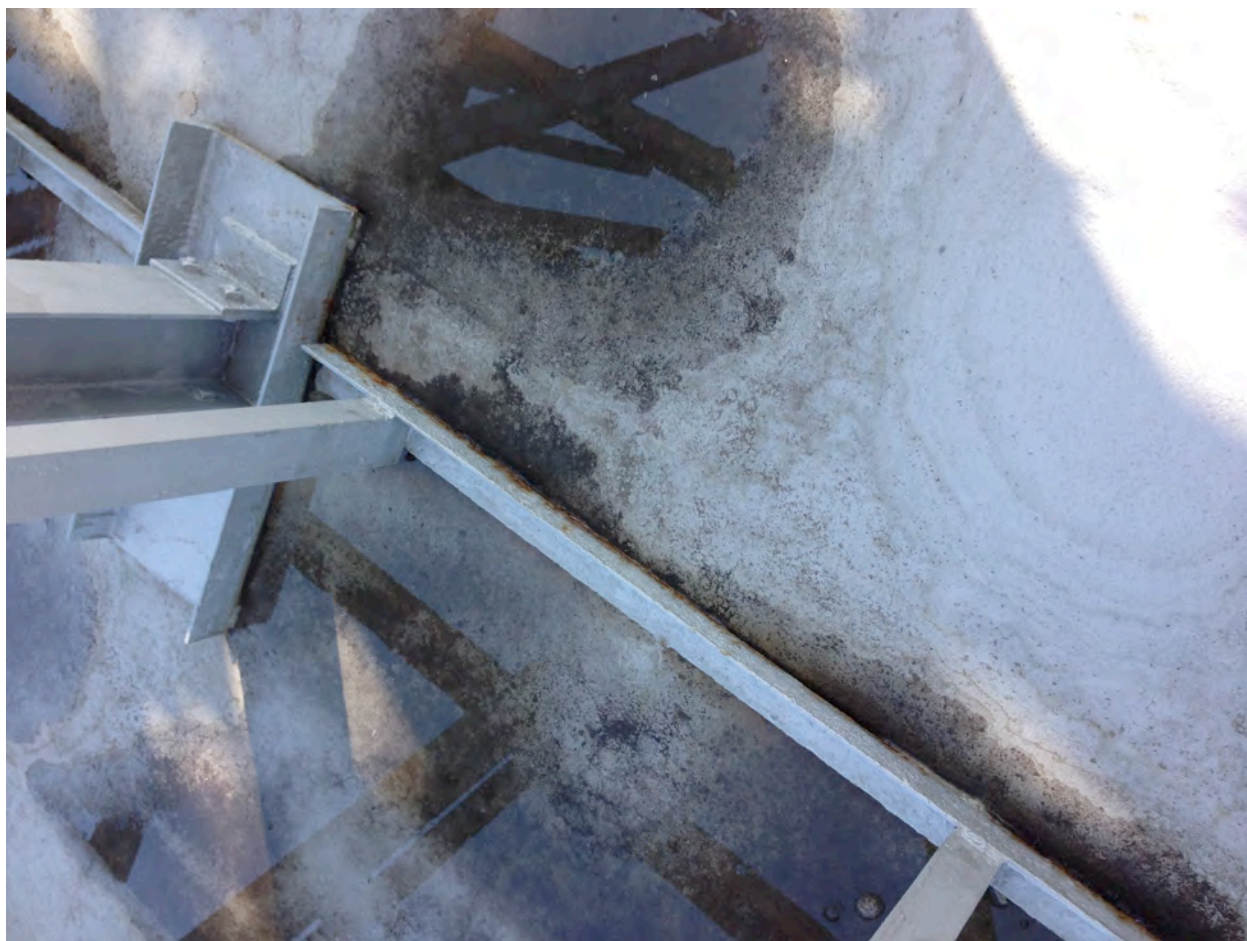
Mezzanine Pooling Water & Sediment
