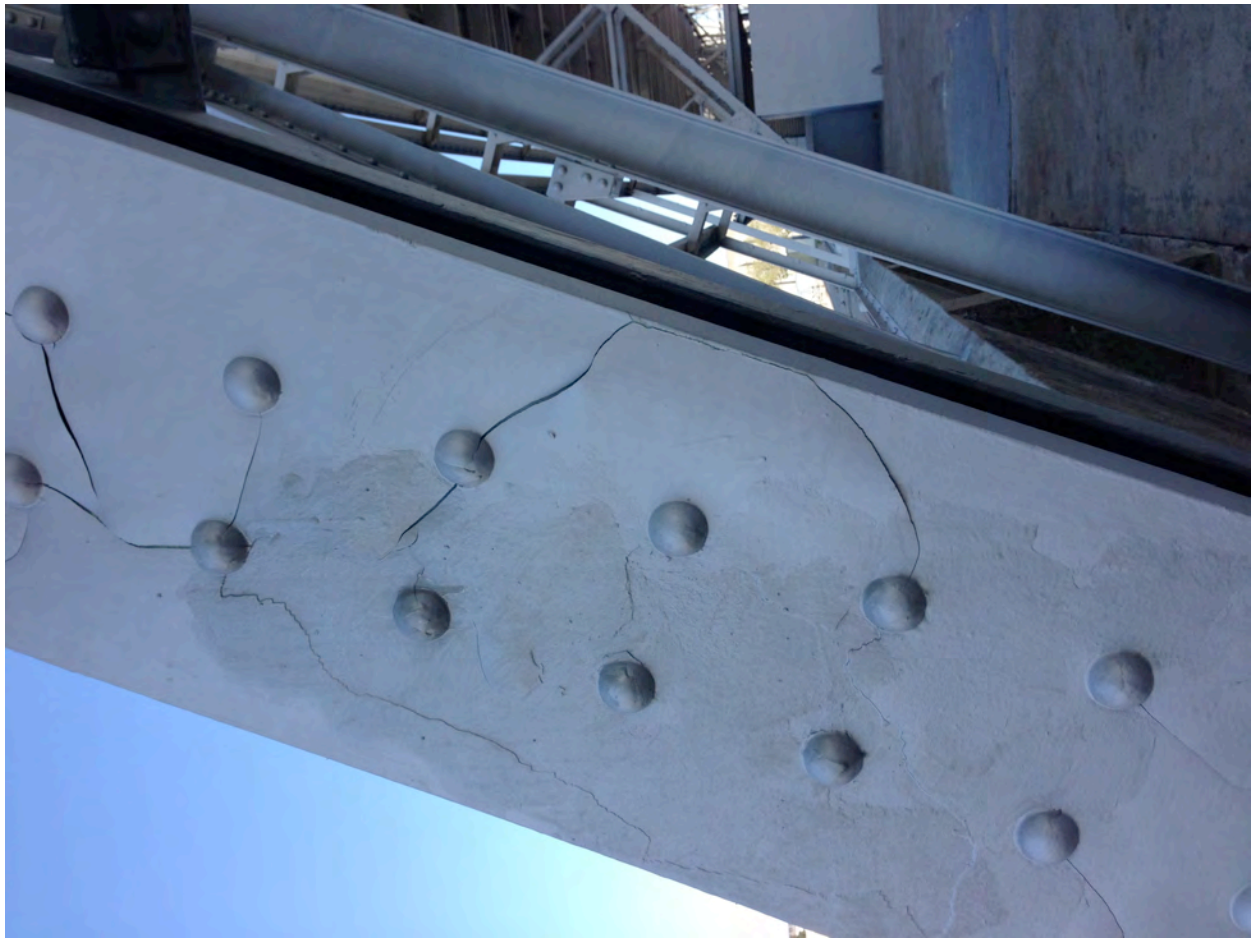
Delaminating encapsulant and original paint, vertical steel
