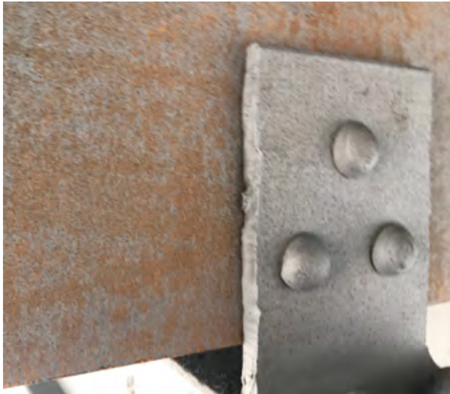
Photograph 9 – Tight-tolerance mated flange/beam connection after removal of paint/coatings with media blasting. (Note: the brown areas in the photo correspond to areas of rust formation due to the wet decontamination of the abated steel)
