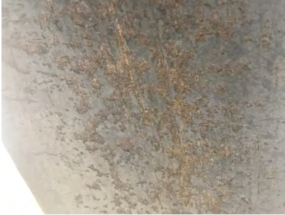
Photograph 2 – Mill scale present on structural steel after paint/coating removal with UHPW system.
