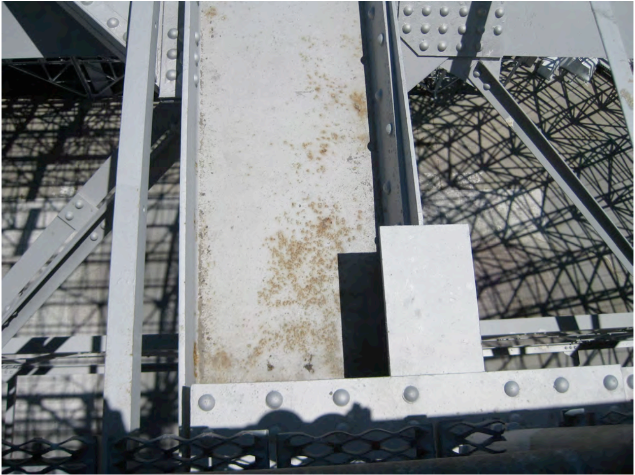
Roof-top rusting of NTCRA Coating
