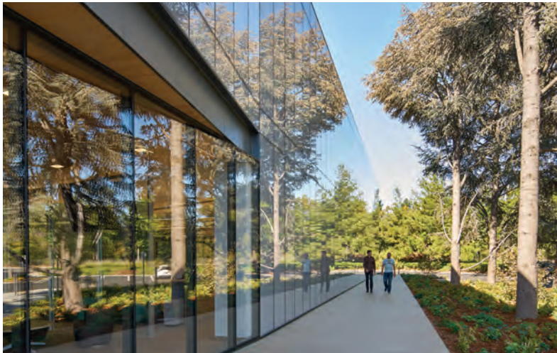
Glass Curtain Wall
