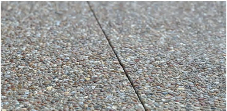
Seeded Aggregate Cast-in-Place Concrete
