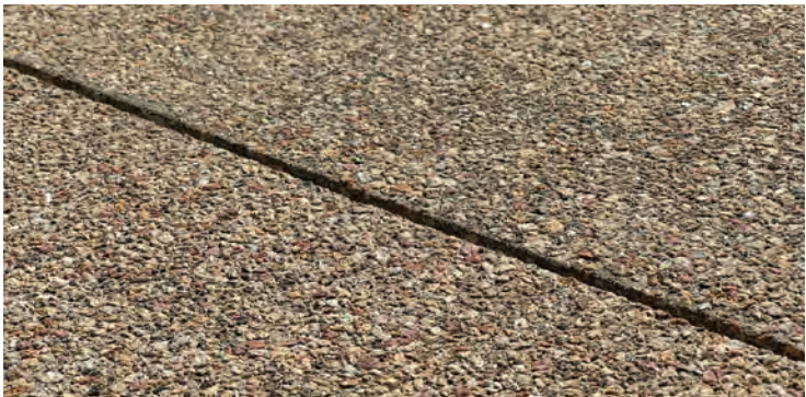
Exposed Aggregate Cast-in-Place Concrete
