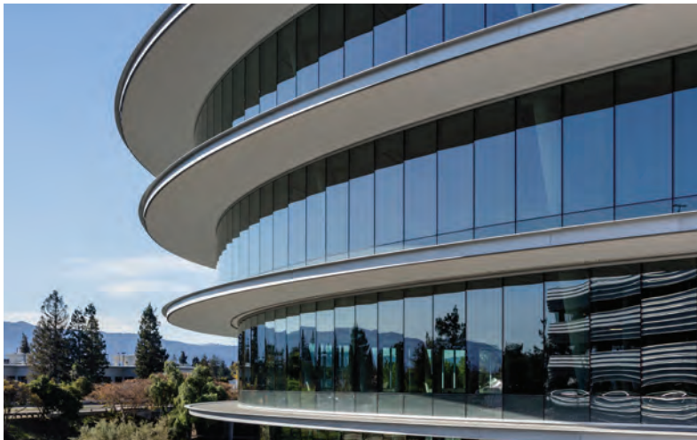
Plaster Soffit, Metal Fascia
