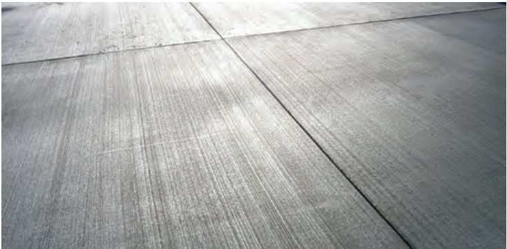
Smooth Cast-in-Place Concrete
