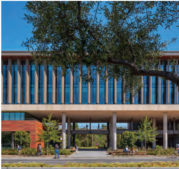
Utilizing Facade Depth to Shade Glazing
