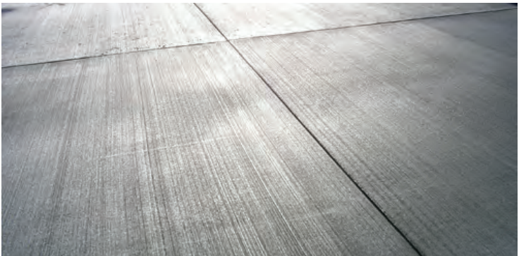
Smooth Cast-in-Place Concrete
