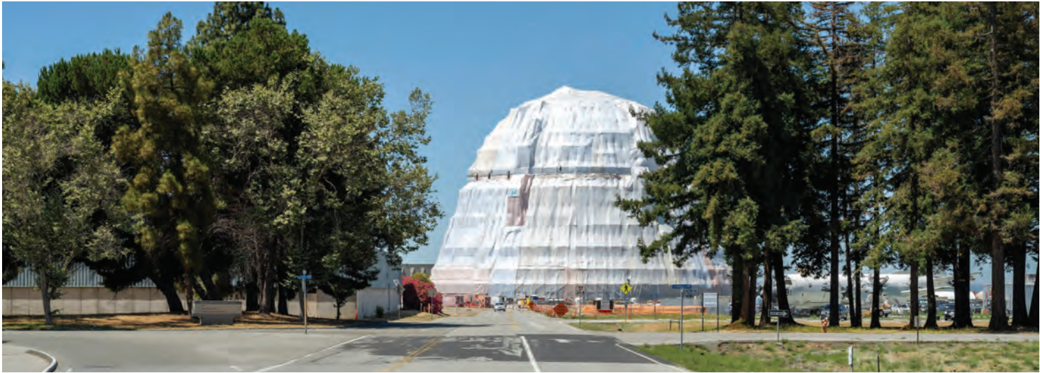
8 Site Frontage: View from Existing Cody Road towards Hangar One
