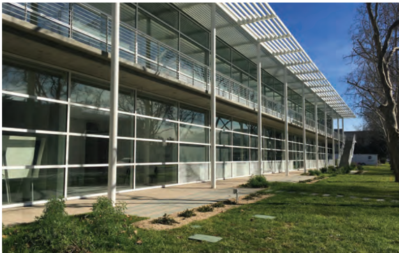
Cast-in-Place Concrete, Glass Curtain Wall, Painted Structural Steel
