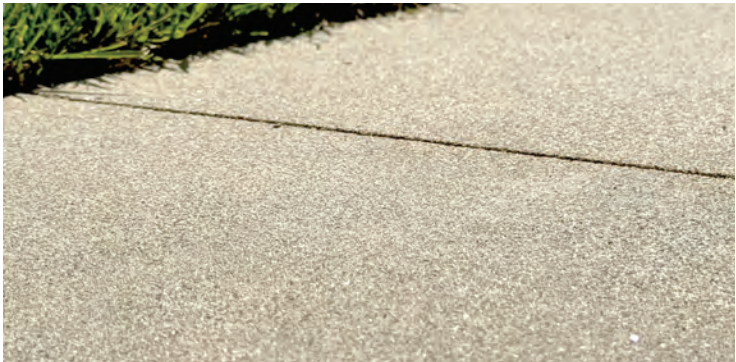
Exposed Aggregate Cast-in-Place Concrete
