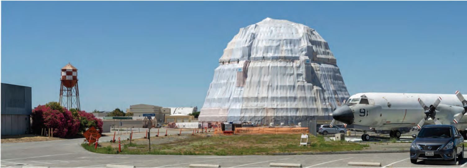
7 Site Frontage: View from Realigned Cody Road towards Hangar One
