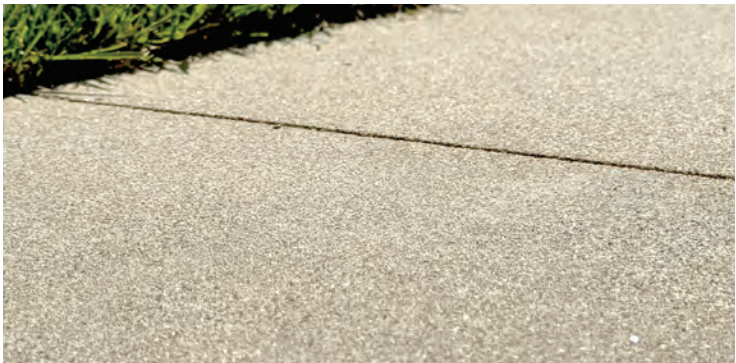
Exposed Aggregate Cast-in-Place Concrete
