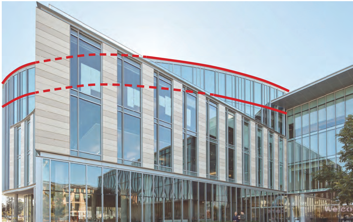
Vertical Extension of Building Facade, Integral to Building Form
