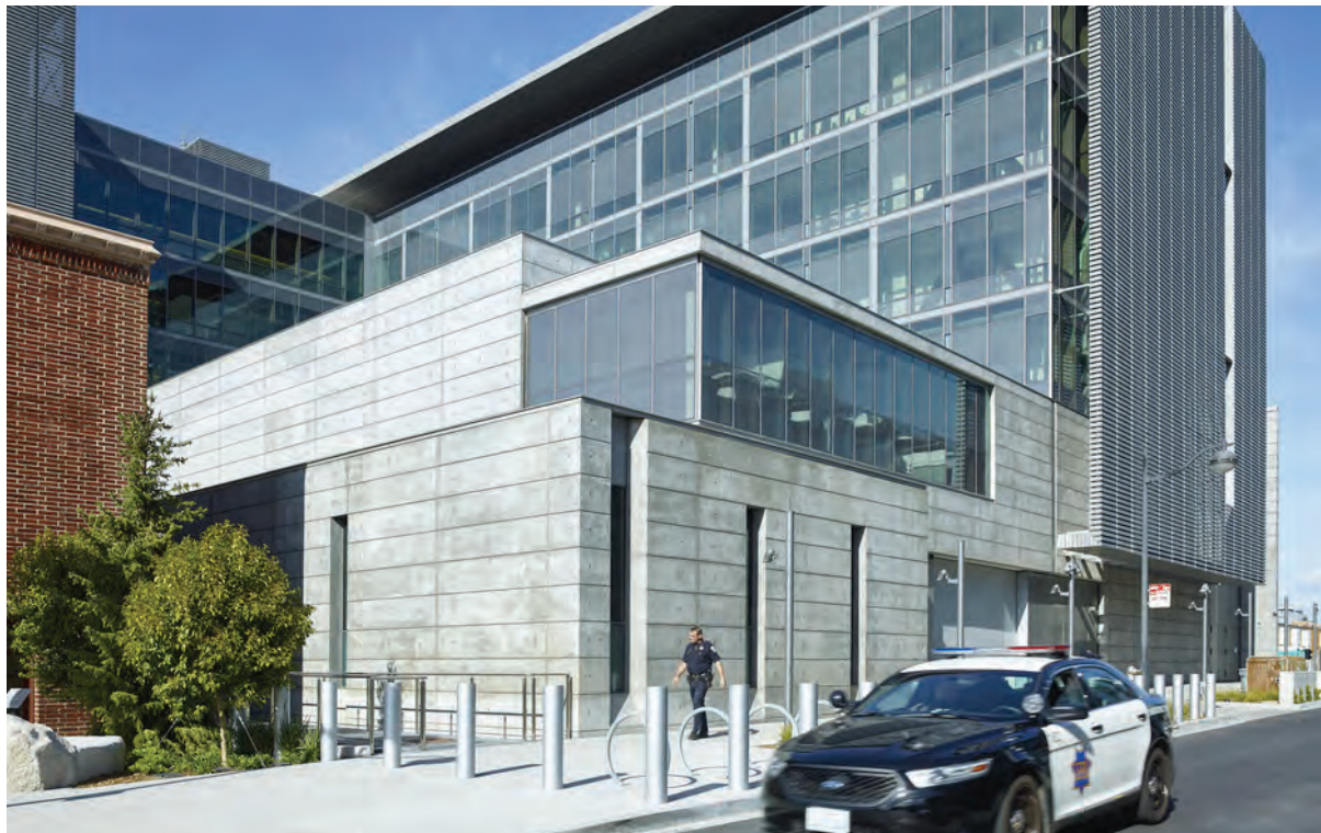
Recessed Service Entry Designed as Part of the Building Facade
