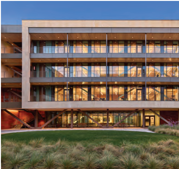
Utilizing Facade Depth to Shade Glazing
