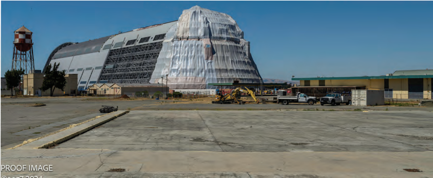
3 Site Frontage: View towards Hangar One
