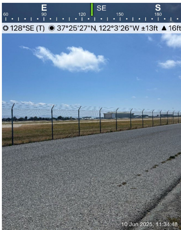
Photo 11 – Security fence along Zook Road.
