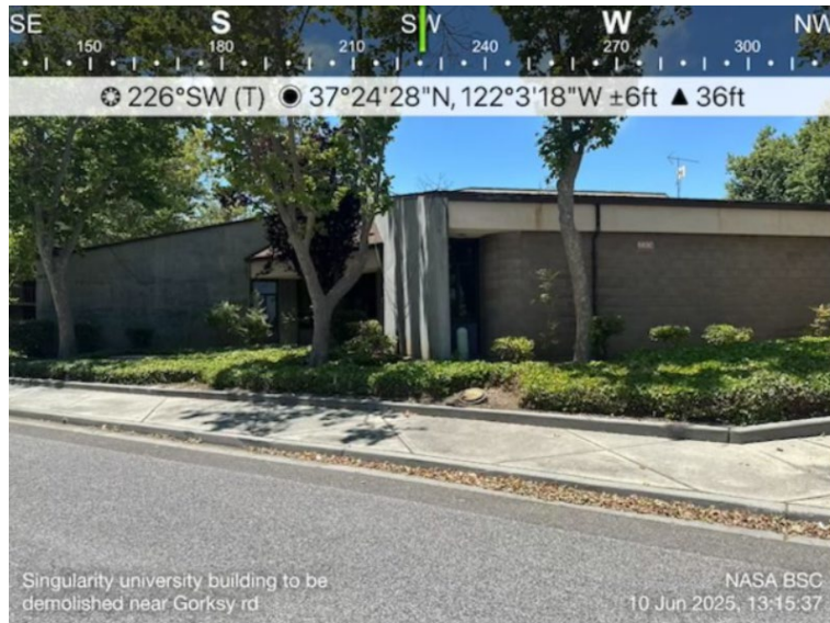
Photo 19 – Building to be demolished near Gorsky Road.
