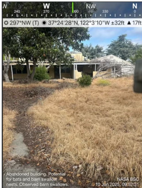
Photo 6 – Vacant buildings within developed land cover.
