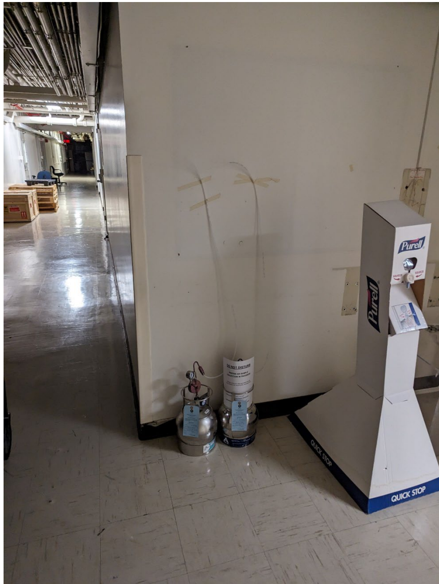
N213-B-08-OFF & N213-B-08-OFFD Building N213, V001 Elevator Vault January 14, 2024
