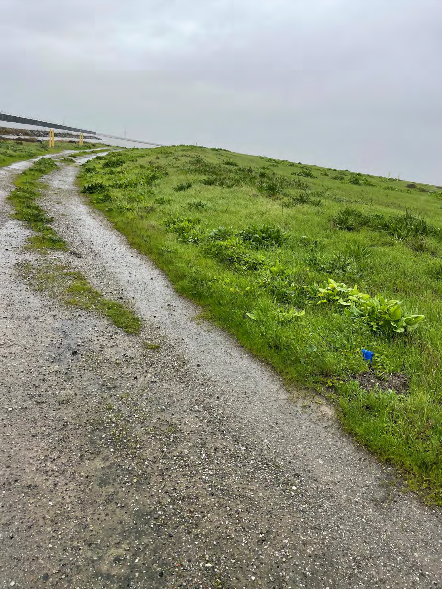
Photo 3: Site 1 – Facing North – West edge of cap along perimeter road.
