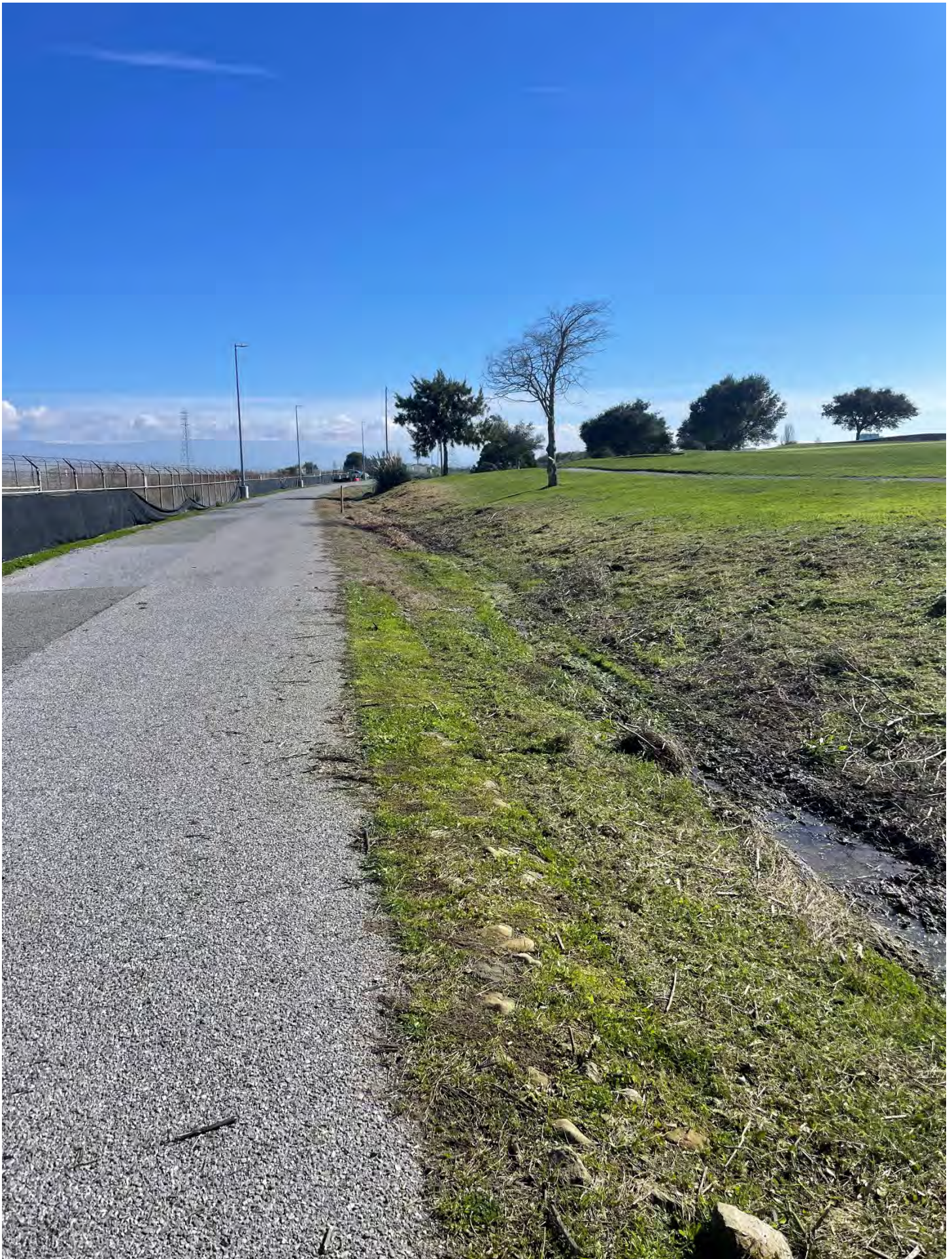
Photo 13: Site 22 – Facing East – Drainage swale and slope vegetation cleared on February 9, 2024.
