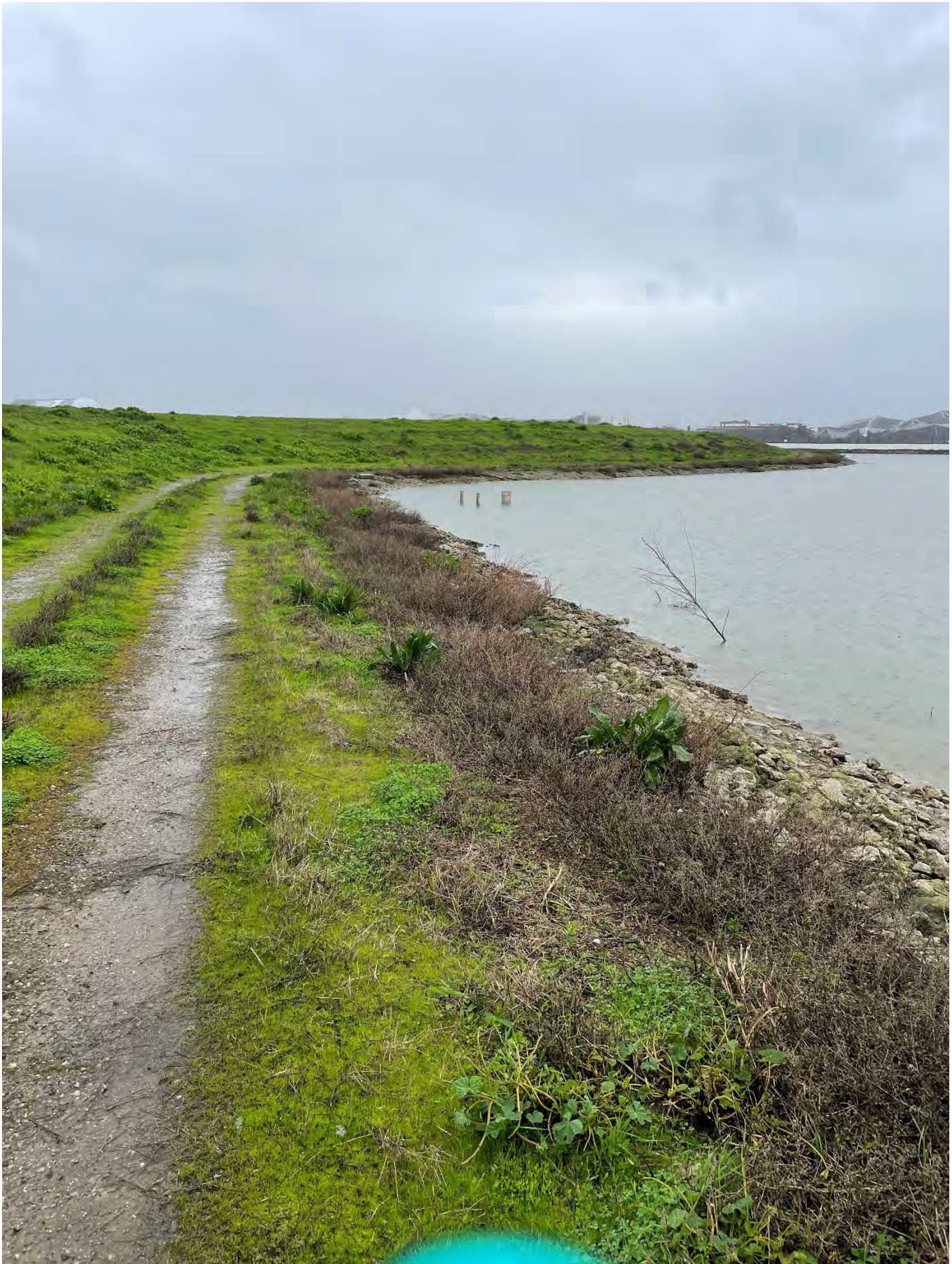
Photo 4: Site 1 – Facing West - North slope of landfill along perimeter road.
