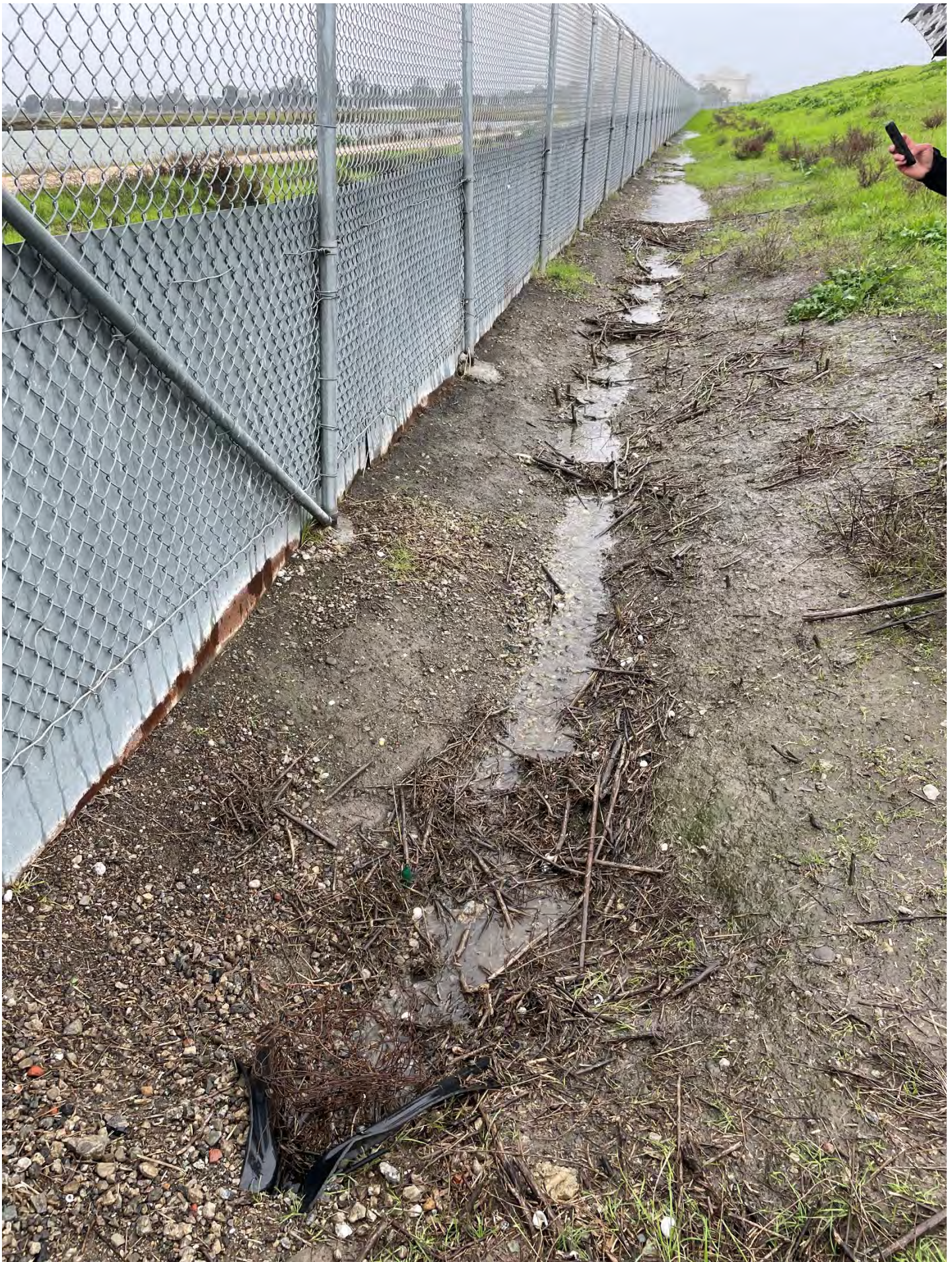
Photo 5: Site 1 – Facing south – Eastern slope and drainage channel along fence-line.
