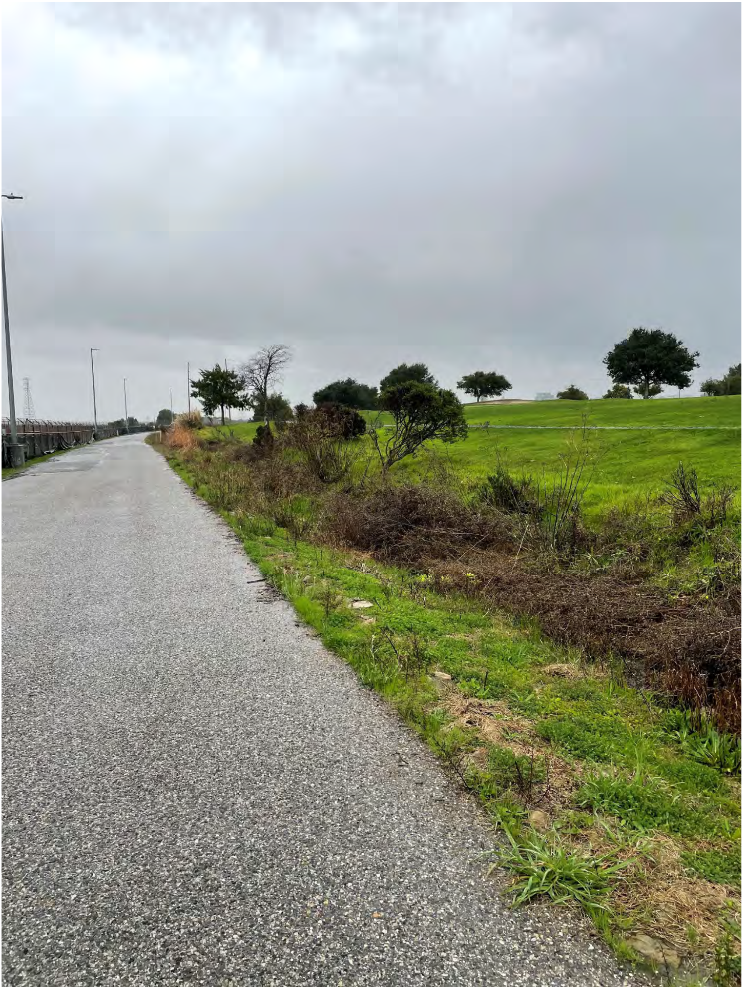
Photo 12: Site 22 – Facing East – Drainage swale along perimeter road.
