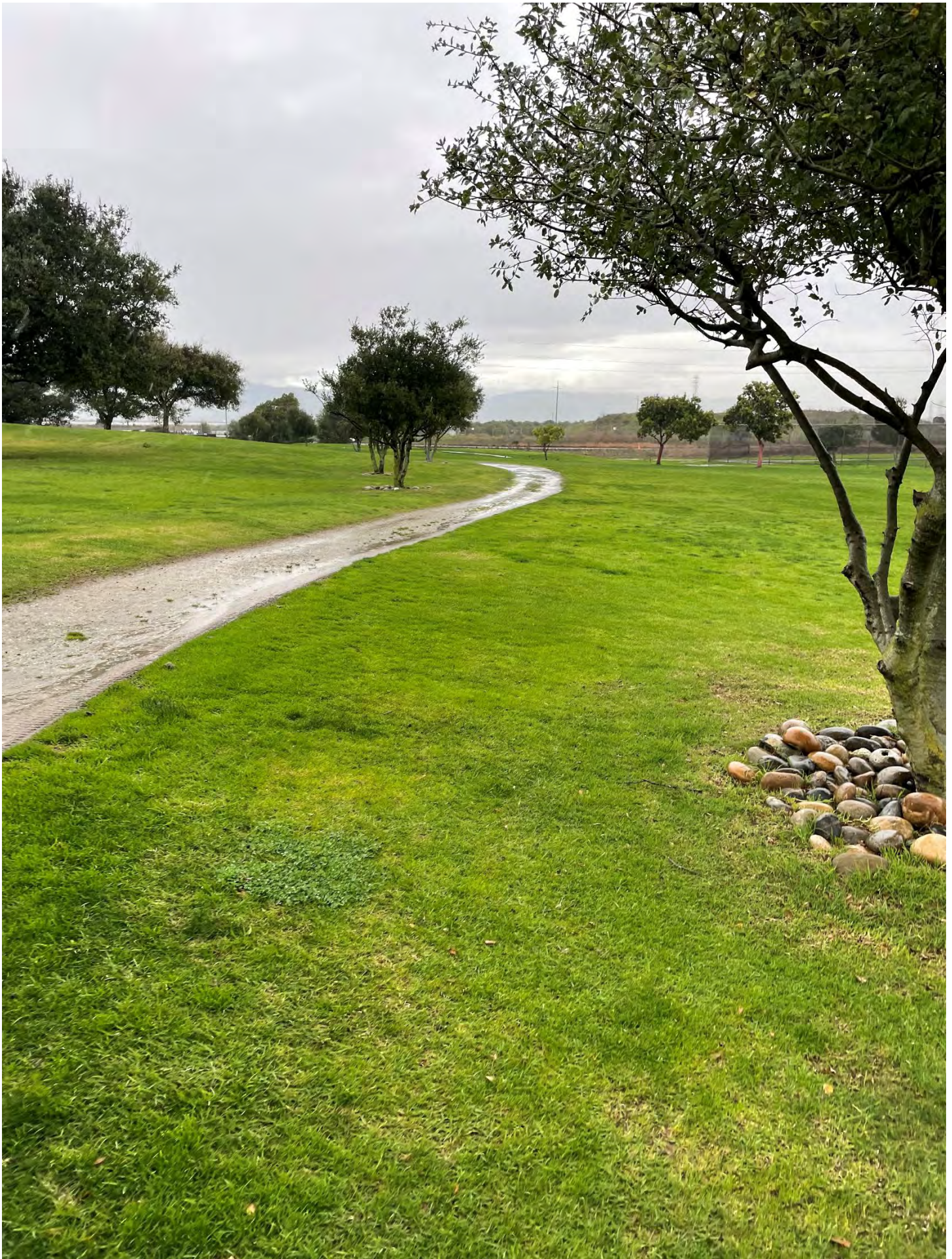
Photo 11: Site 22 – Facing East – Eastern portion of cap showing tree wells and cart path.
